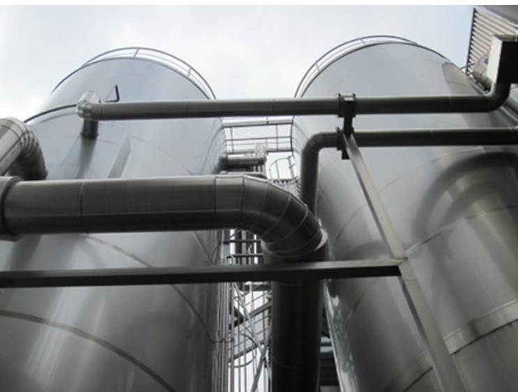
PIC LEFT ice silos with 5000 kWh storage capacity each PIC RIGHT ice maker for 6 to/h. At 10 h buildup time 5600 kWh
